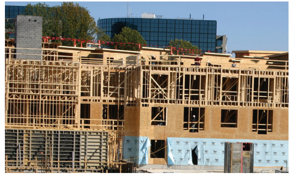
Figure 10—Type V construction
