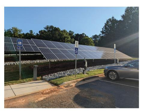
Additions must meet the new construction requirement for renewable energy systems based on the square footage of the addition alone. This PV system, installed at ASHRAE's headquarters in Georgia, was a key strategy for achieving net zero energy in an existing building.
