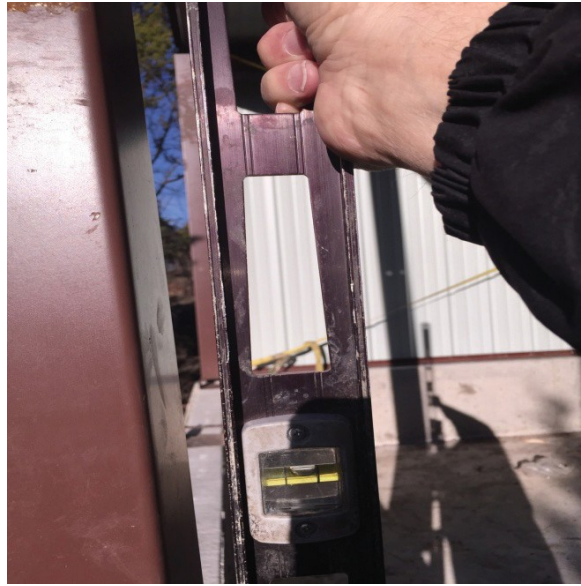
Figure 3.2-1: Non-Acceptable Vertical Tolerance
