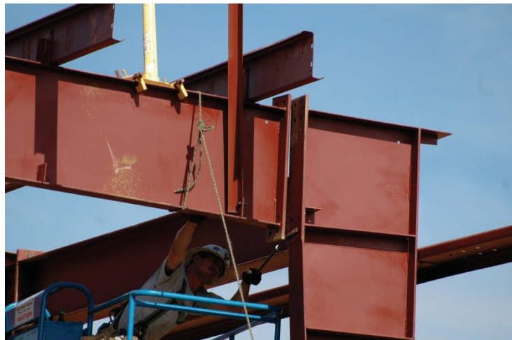
Figure 3.5-1: Bolted End-Plate Connection
