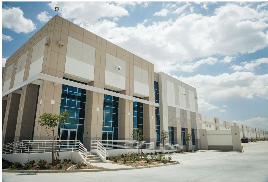
Large concrete and steel buildings can be difficult to send a signal through. A booster may be required. (Photo courtesy of Erik Isakson/Tetra images via Getty Images)
