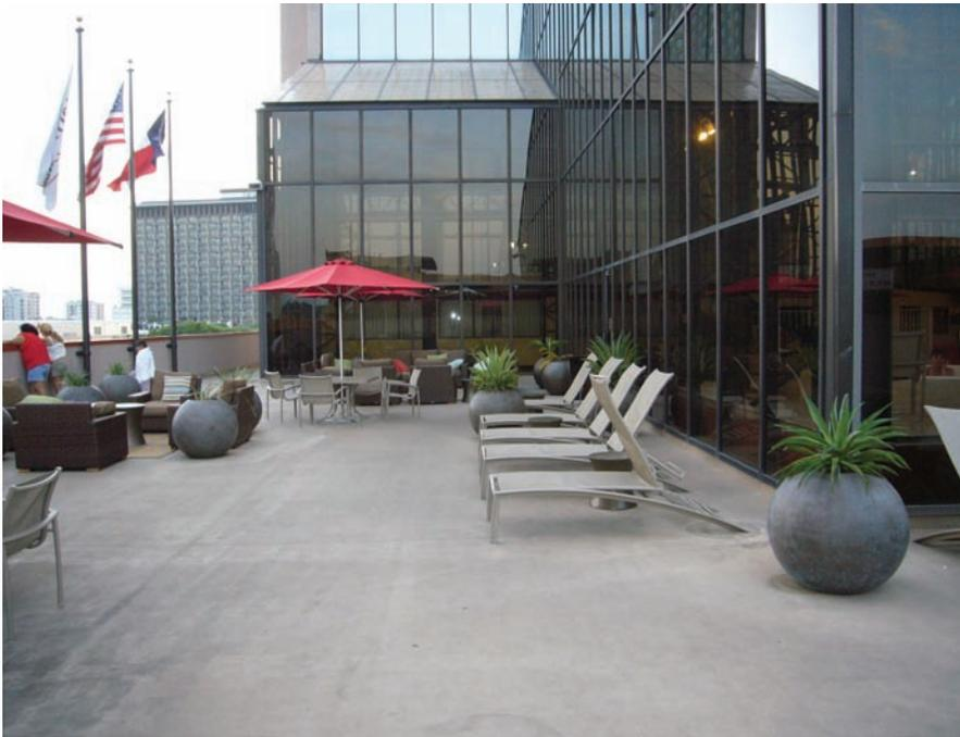
A landscaped roof. The roof is a concrete deck, which is classified by the IBC as a Class A roof covering.
