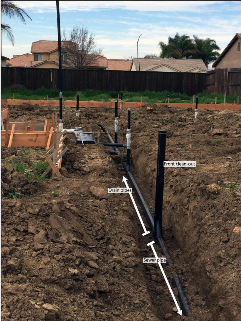
**IDENTIFYING DRAIN PIPES FROM SEWER PIPE**
