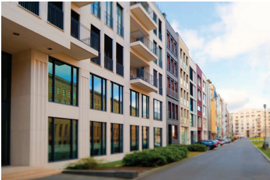
Photo courtesy of PPAMPicture
