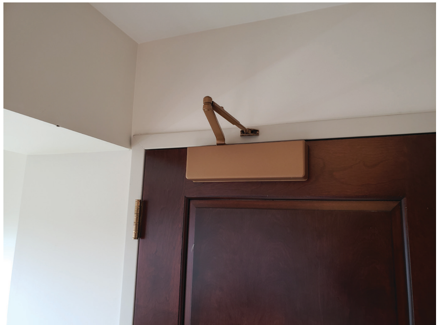
FIGURE 2-1 Door from garage to dwelling does not need self-closing device
