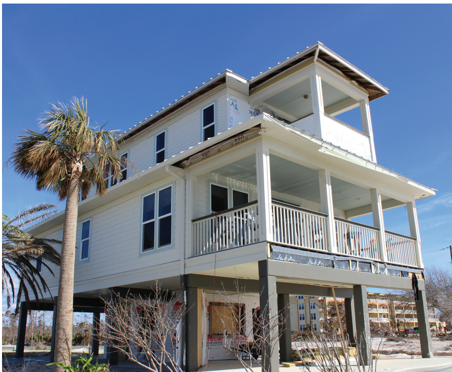
Failure of soffit due to Hurricane Michael
