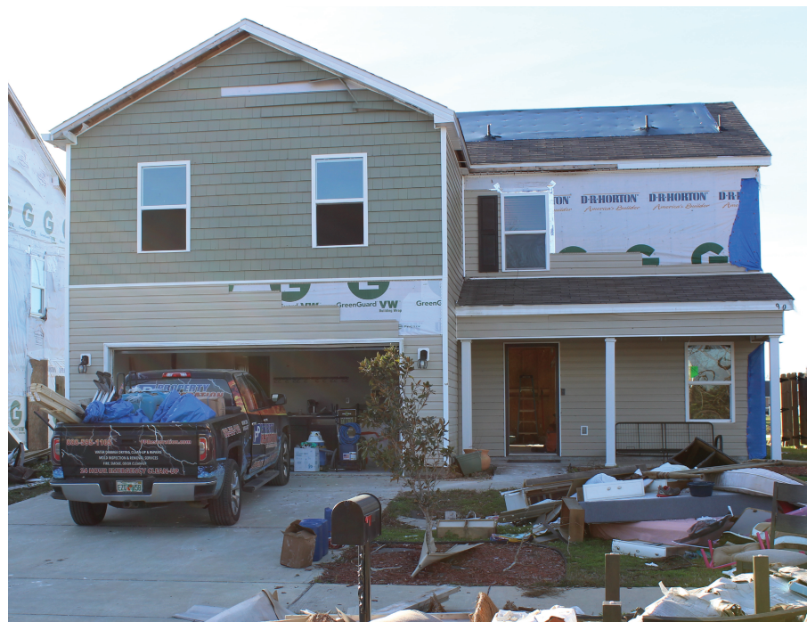
Failure of vinyl siding and soffit due to Hurricane Michael
