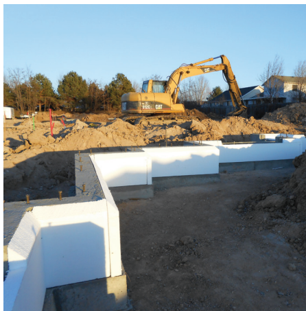
Frost-protected shallow foundation
