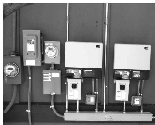
Figure 6: Example String Inverter
