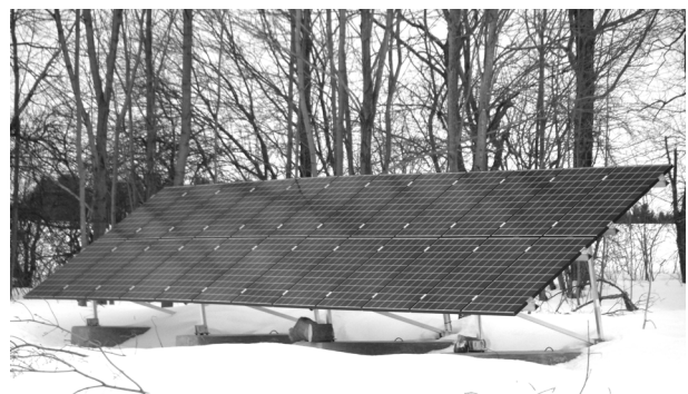
Figure 2: Example Groundmount PV
