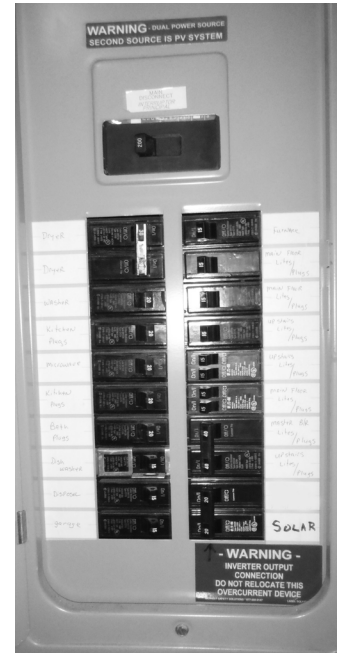
Figure 10: Back-fed Breaker Location
