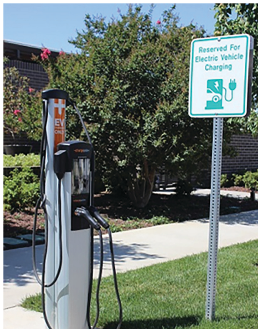
FIGURE 2 State Housing Law Program staff photo: electric vehicle charging station at multifamily residential complex.
