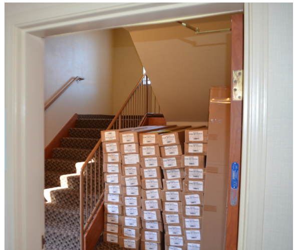
FIGURE 3-1 Ignition of combustible materials beneath the egress stairs can eliminate the stairs as an escape path, and therefore storage in that location is a violation of the IFC.
