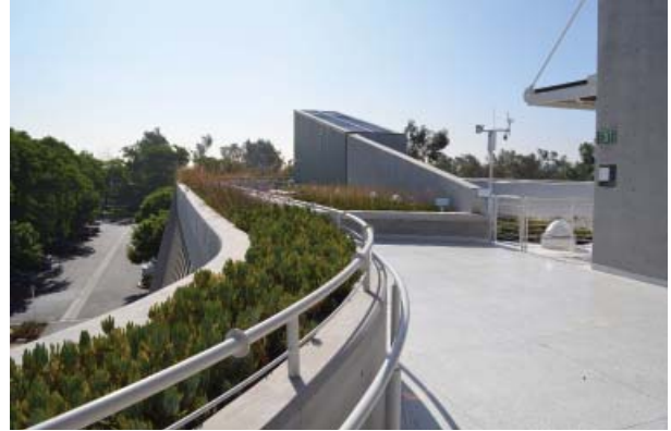
FIGURE 3-14 Landscaping on the roof must be maintained in a safe condition and allow fire-fighting access.
