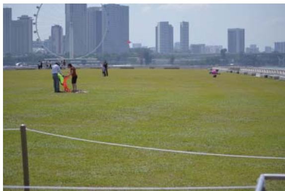
FIGURE 3-13 This grass-covered roof provides a park-like area for recreation.
