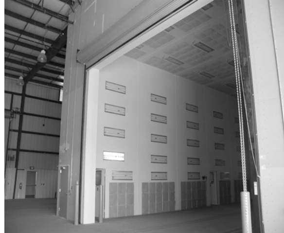
Figure 3-1: Group H-2 Spraying Room
