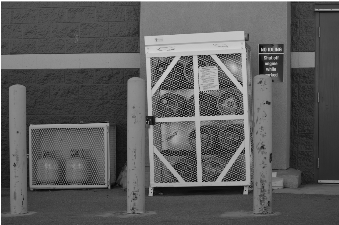
Forklifts operated inside this building are driven outside to replace the empty LP-gas cylinder with a full cylinder.
