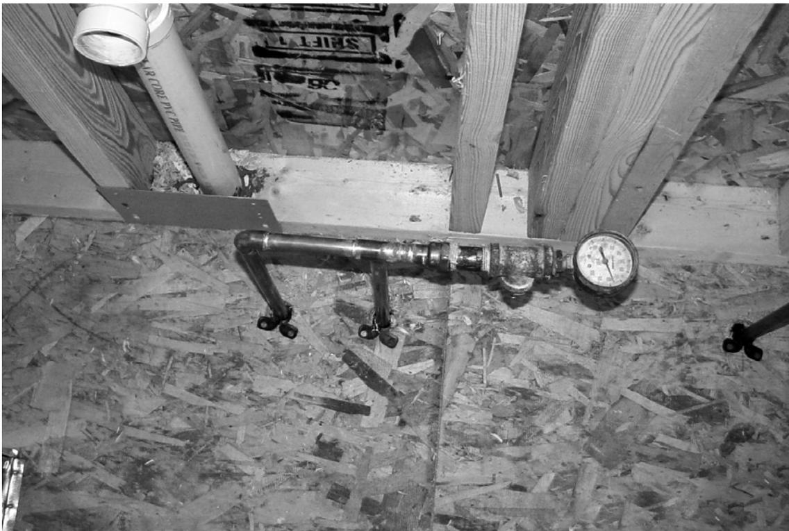
Testing with air is not permitted on plastic piping systems because of the hazards of a sudden release of energy, which could cause a separated piece of piping or a fitting to become a projectile causing serious injury.
