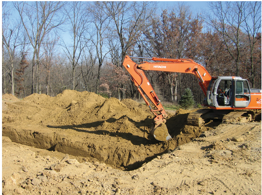
Figure 3-4 Excavation for foundation of a detached dwelling.
