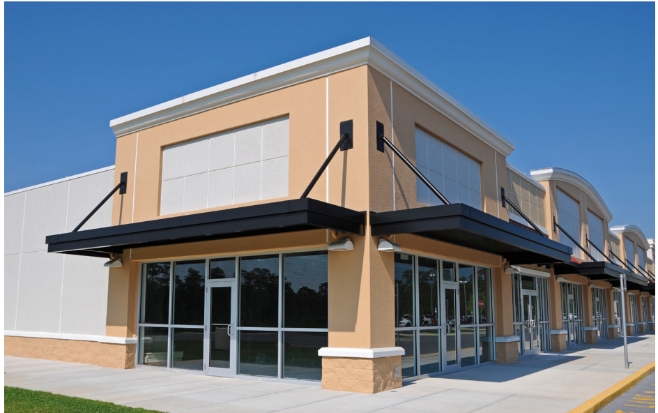
FIGURE 3-1 Commercial shopping center.
