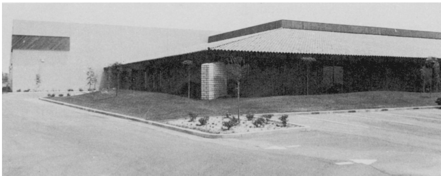
Figure 1.2a Foreground: Office portion of wood-frame construction. Background: Warehouse with concrete tilt-up walls and wood roof system. (Photo courtesy of Mike Hausmann.)
