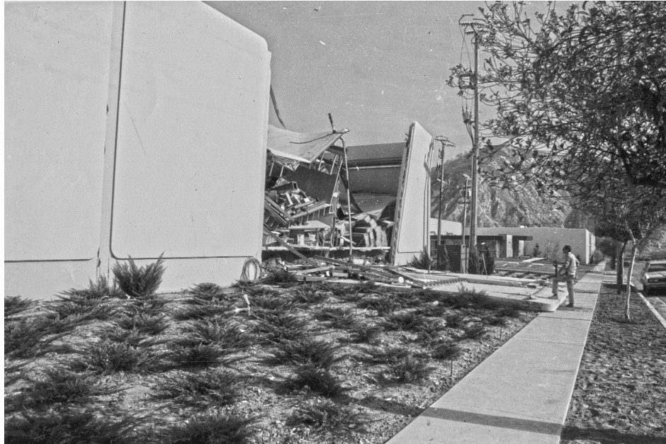
Figure 1. Damage from the 1971 San Fernando Earthquake, Feb 9, 1971
