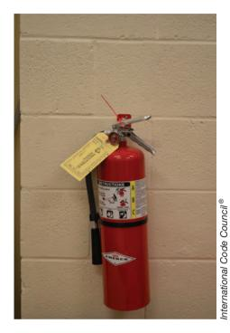
Where each classroom in a Group E occupancy is provided with a fire extinguisher, additional fire extinguishers in the corridors are not required.
