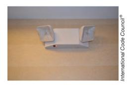
Emergency egress lighting is manually tested monthly unless equipped with self-testing and self-diagnostics.
