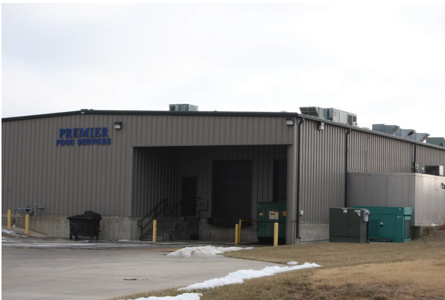
Commercial catering facility
