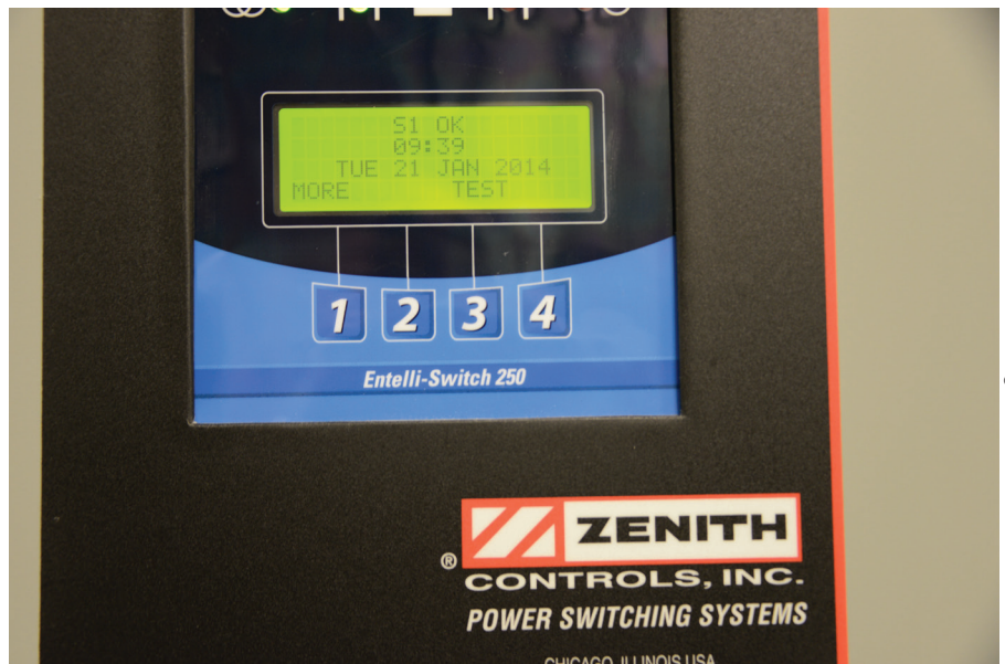
Power switching (load transfer) system in hospital
