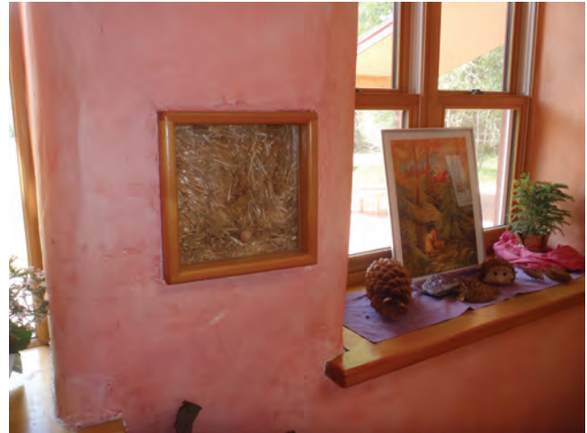
FIGURE 3-7 Straw bale insulation
