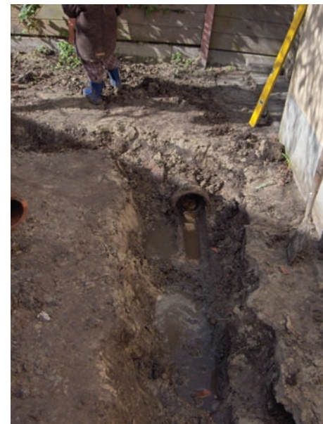
FIGURE 1-8 A leaking sewage system would require repair under the provisions in the IPMC
