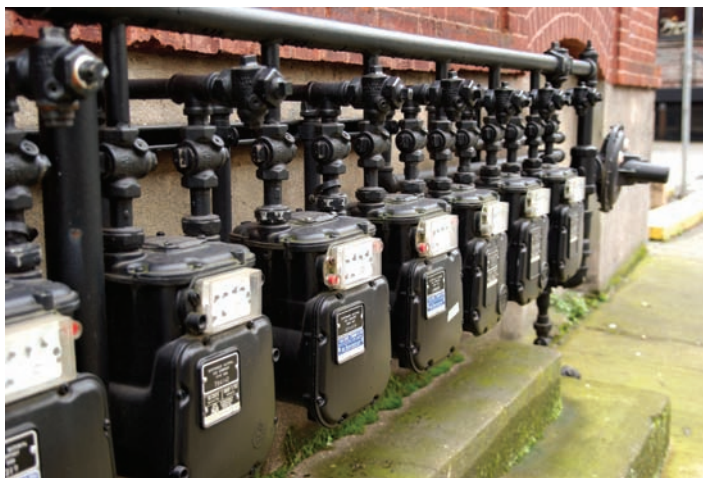
FIGURE 1-7 Natural gas meters. The piping on the discharge side of each meter is regulated by the IFGC
