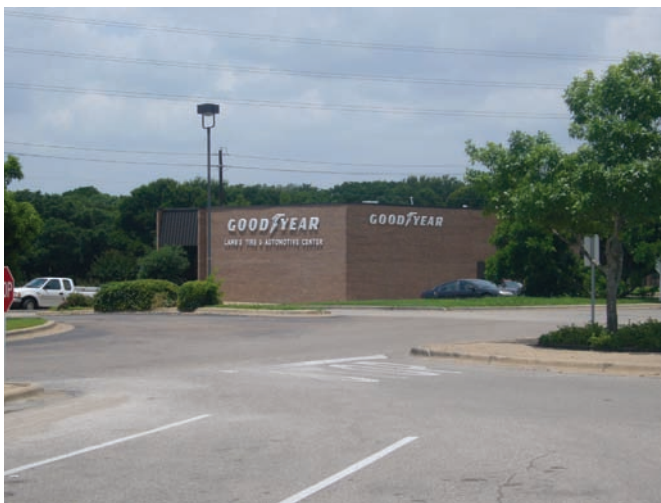
FIGURE 1-3 IBC regulated building
