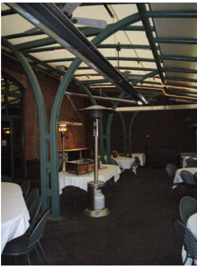
FIGURE 1-10 Two portable outdoor gas-fired heaters used inside a building. Based on the requirement in Section 102.1, item 2, a fire inspector would cite this installation as a violation of the requirements in Section 603.4.2.1.1
