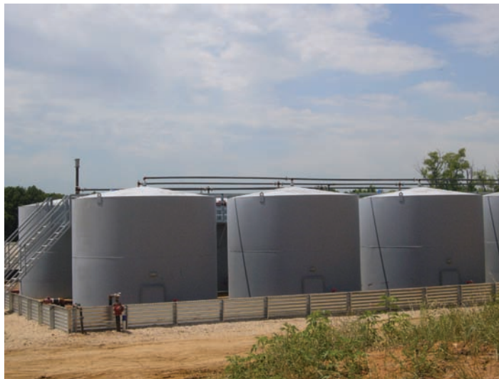
FIGURE 1-13 The design of these petroleum storage tanks was required by the fire code official to comply with one of the atmospheric storage tank design and construction standards developed by the American Petroleum Institute
