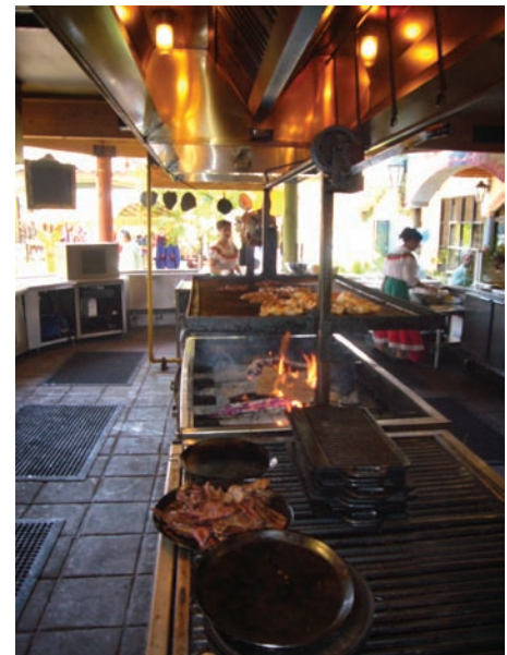
FIGURE 1-6 A commercial kitchen cooking system is regulated by the IMC and IFGC. If the appliances are supplied by fuel gas, the system is also regulated by the IFGC
