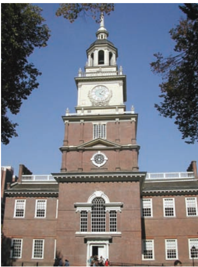
FIGURE 1-12 Historic buildings must comply with a fire protection plan approved by the fire code official
