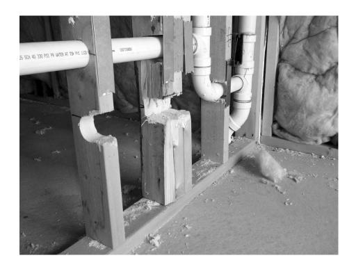
The International Building Code (IBC) and the International Residential Code (IRC) limit the amount of notching and boring of wood framing members to preserve the integrity of the framing system.
