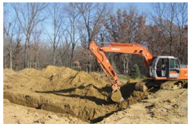
FIGURE 3-4 Excavation for foundation of a detached dwelling
