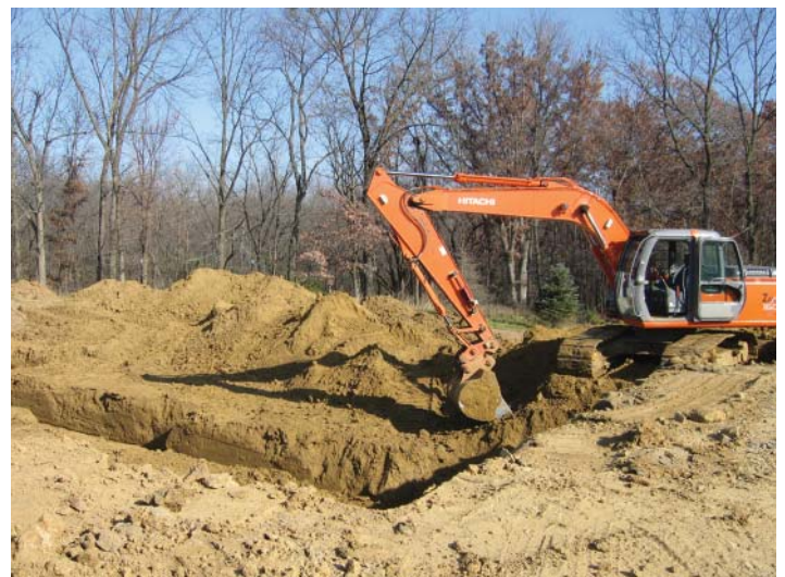
FIGURE 3-4 Excavation for foundation of a detached dwelling
