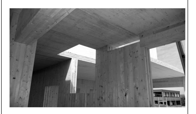
Cross-laminated timber floors regulated as Type IV heavy-timber construction must be continuous from support to support and mechanically fastened to one another. Unlike sawn or glued-laminated plank floors, CLT is permitted to be connected to walls without a shrinkage gap if swelling or shrinking is considered in the design.
